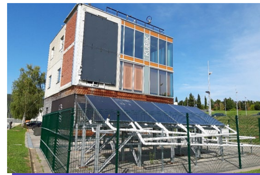
Figure 21: KUBIK facilities at Derio (Bizcaia, SPAIN)
